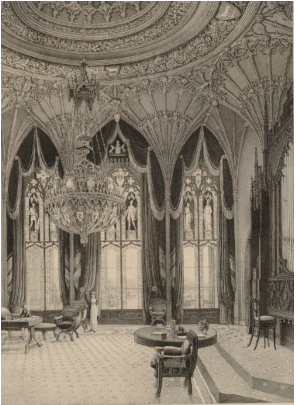
Figure 2. The saloon at Eaton Hall in 1826 with part of William Porden's Gothic organ case just visible on the right.
